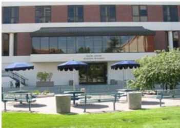
Ansari Business Building (# 063)
